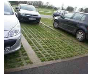
Typical Precast Concrete Paving Layout
